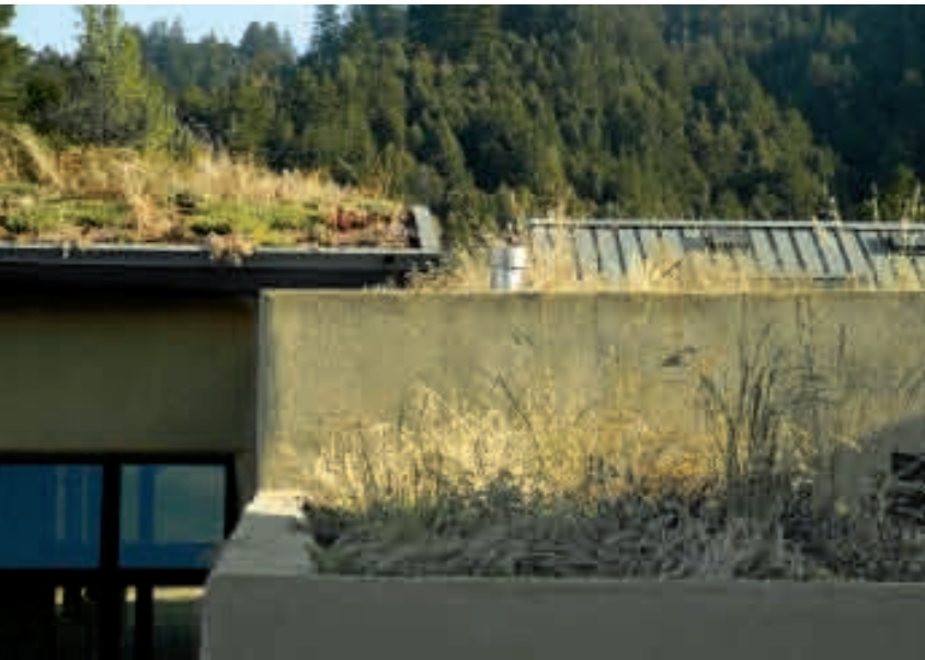
LEFT: The dining hall of the Presentation Retreat & Conference Center in Los Gatos, designed by Berkeley-based Daniel Smith & Associates, is a straw-bale building with a green roof and solar panels.
